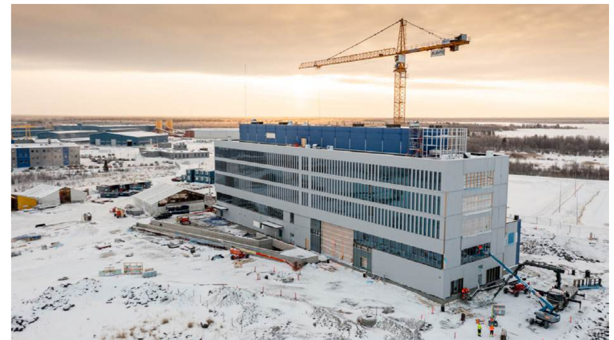
The administration building was quite far along. Photo courtesy of Fennovoima
